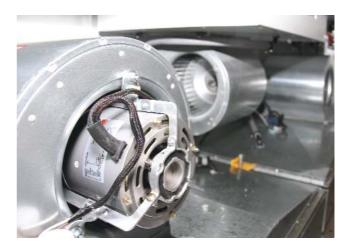
**Fans.** Separate direct-drive fans are provided for the exhaust and laminar flow HEPA filters. Fans are fitted with speed controllers to enable airflows to be maintained through filter life.
